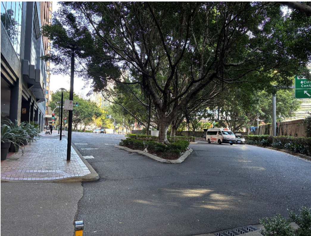
Figure 11. Day Street road reserve, looking south
